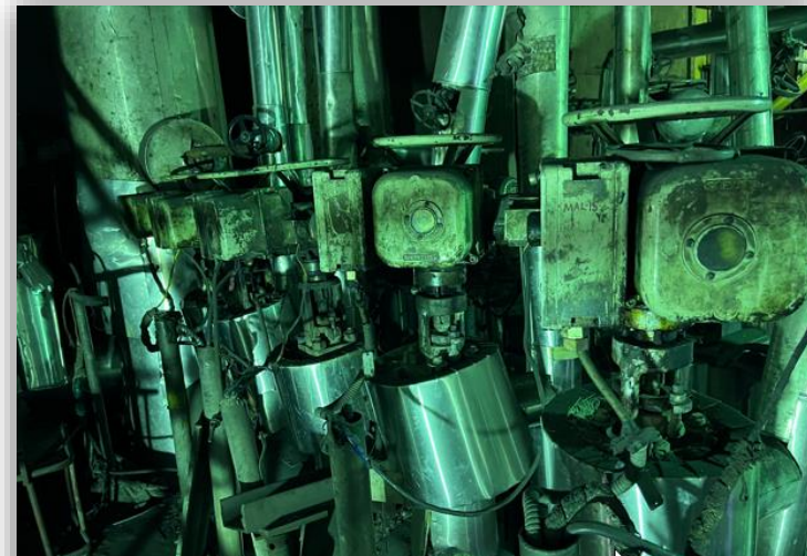
Replace: Turbine Drain Valves
